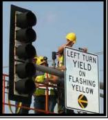
eral benefits from placement of the flashing yellow arrow. The new signal allowed more traffic to move through an intersection, provided additional traffic management flexibility, provided motorists with a clear distinction of yielding to oncoming traffic, and also is a low cost safety measure to help prevent crashes. The FDOT will be in-
